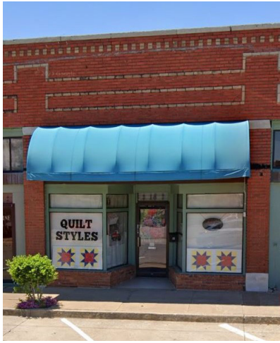
Example of well-preserved bulkheads and display windows in downtown Sapulpa
