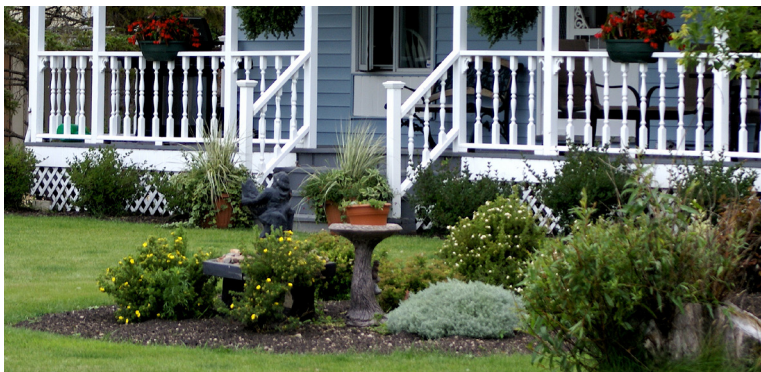
Example of lattice panel foundation enclosure
