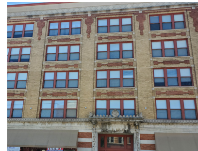
Examples of well-preserved historic windows and appropriately restored windows in downtown Sapulpa
